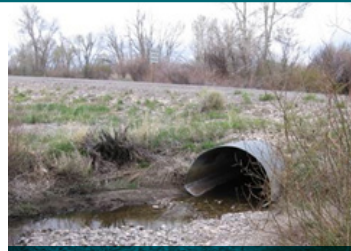
Big Timber Creek Disconnected
