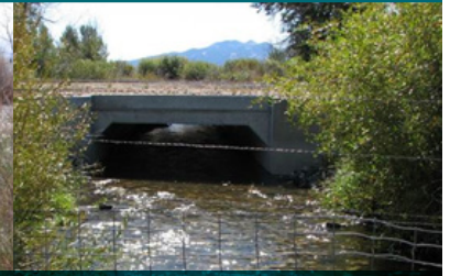
Big Timber Creek After bridge and flow projects
