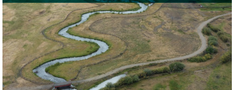
Channel meander project on mainstem Lemhi River
