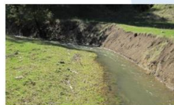
Credit: ODFW Incised channel and trampled vegetation.
